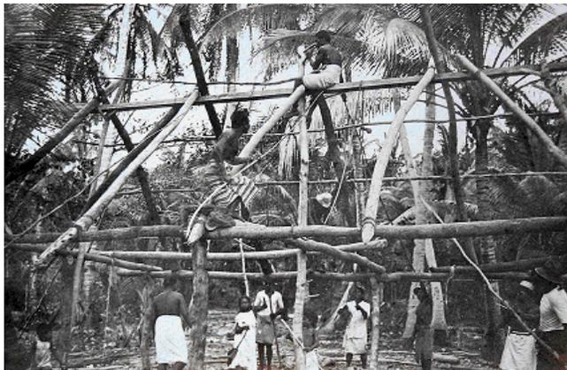
**Figure 1.1: The importance of placement of roofing in *maneaba* structure**
