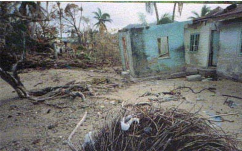
**Photo 3:** House of Tekanabu at Nuku is the house on the beachside opposite Photo 1 (this solid concrete house has also been moved off its foundations by the storm surge from the sea)
